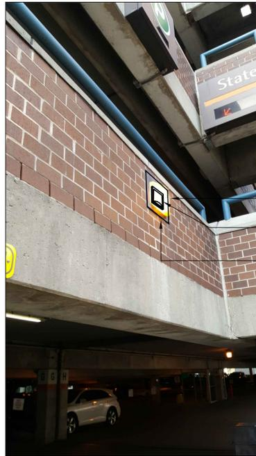
REMOVE EXISTING LIGHT FIXTURE. BACK BOX CAST INTO MASONRY TO REMAIN.
